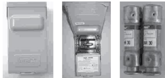
Disconnect switch box for outdoor unit
