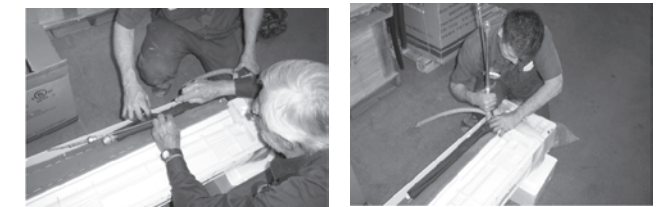
Slice the insulation before bending.
